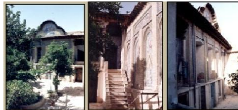
Figure 3. Use of high walls, water and plant and fossette and dragged openings in Atroosh house
