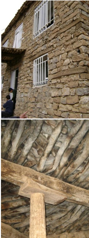
Figures 7, 8: Solid manorary ceiling construction with timber. Hajij village. Resource: authors
